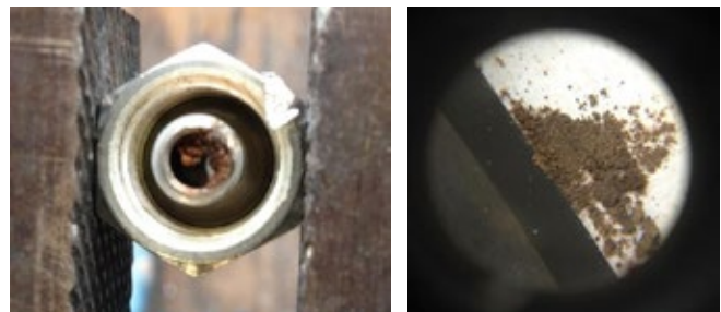
Figure 5: Rust formation due to flame in upstream feed
