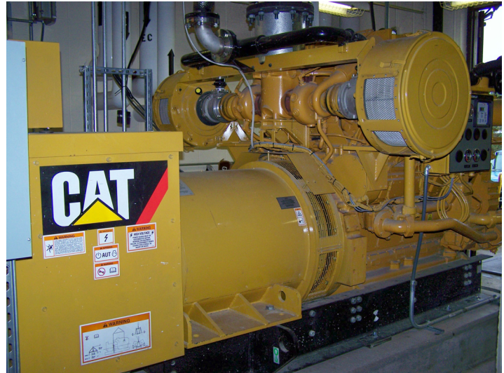
Caterpillar 350kW gas engines powered by biogas at the Gloversville-Johnston treatment plant
