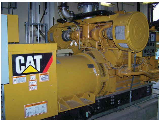
Fig. 2 Caterpillar 350 KW gas engines powered by biogas
